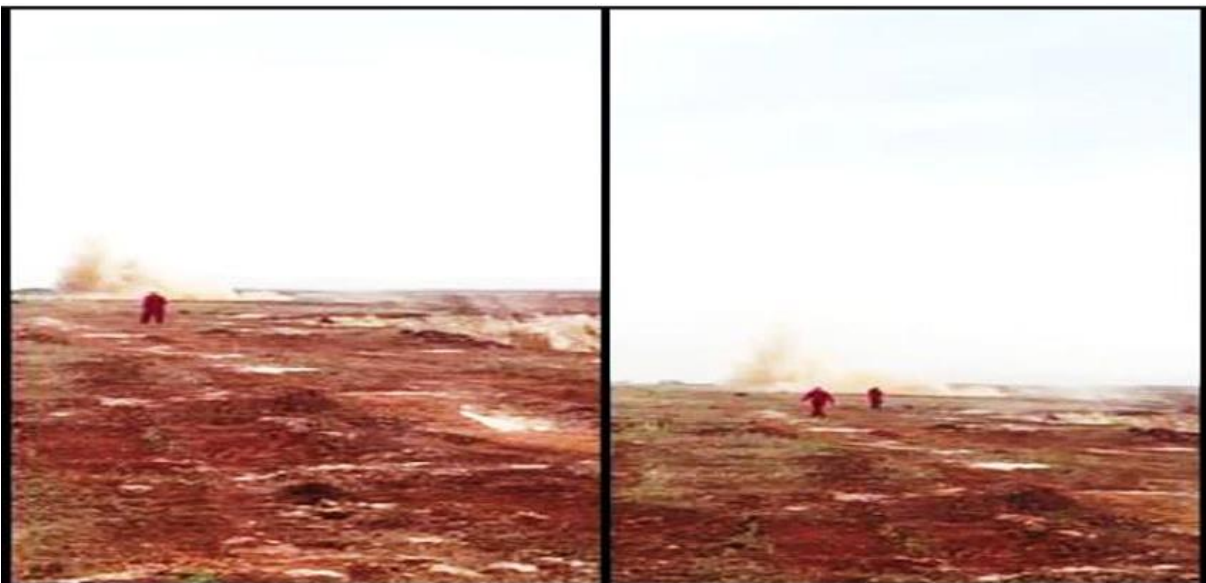
FIGURE 20 : EXECUTION DU TIR
