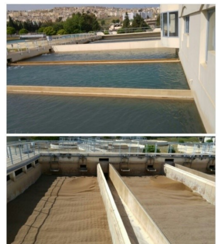
Figure 6:Filtres a sable
