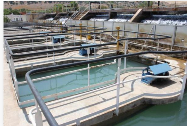
Figure 7: Bassins de coagulation -Floculation
