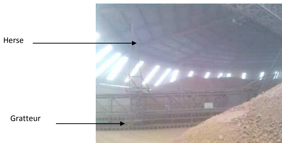
FIGURE 6: HALL DE PRE-HOMOGENEISATION
