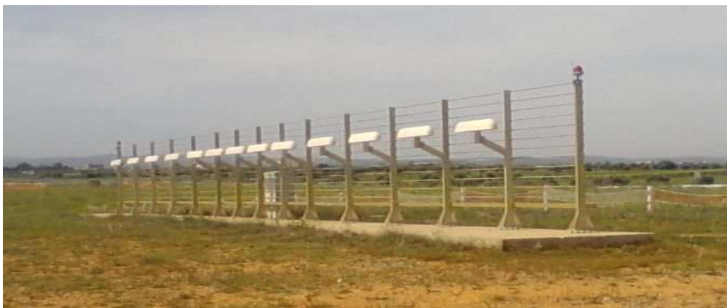
Figure 6: les 13 antennes du Localizer
