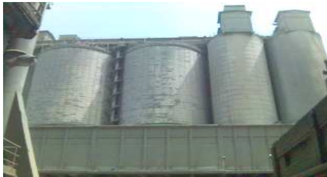
Figure 10 : Stockage du ciment
