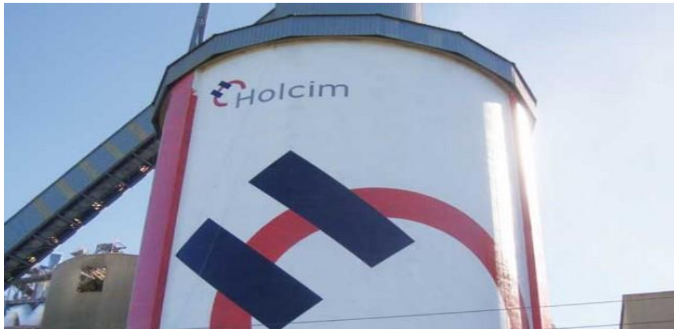
Figure 13: Silos clinker 27300T.
