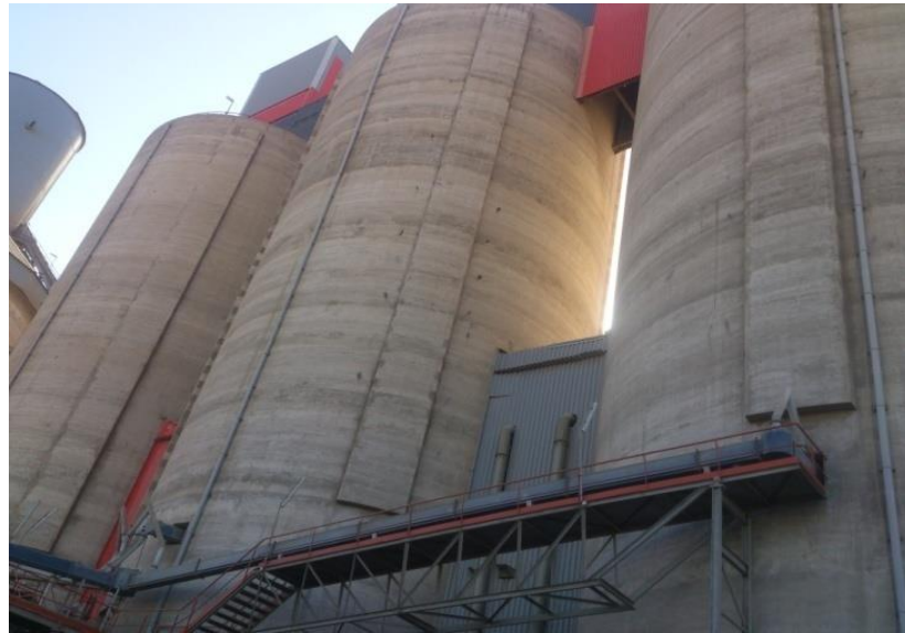
Figure 14: Broyage du ciment.
