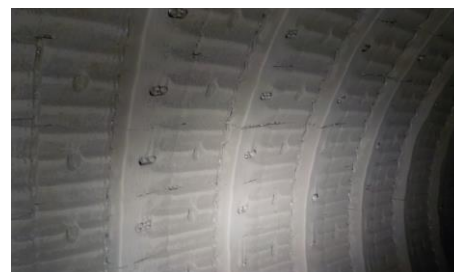
Figure 25 : compartiment 2 blindages classant
