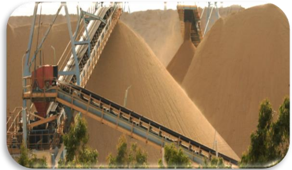
Figure 11: Parc de stockage
