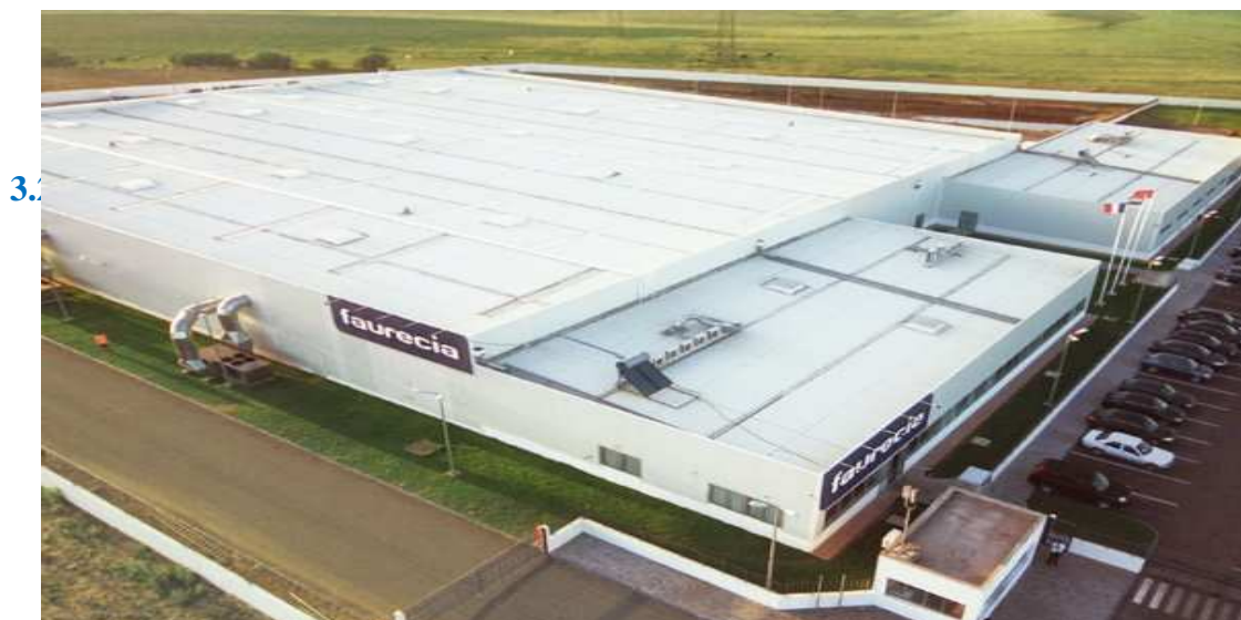
Figure 5: photo du site
