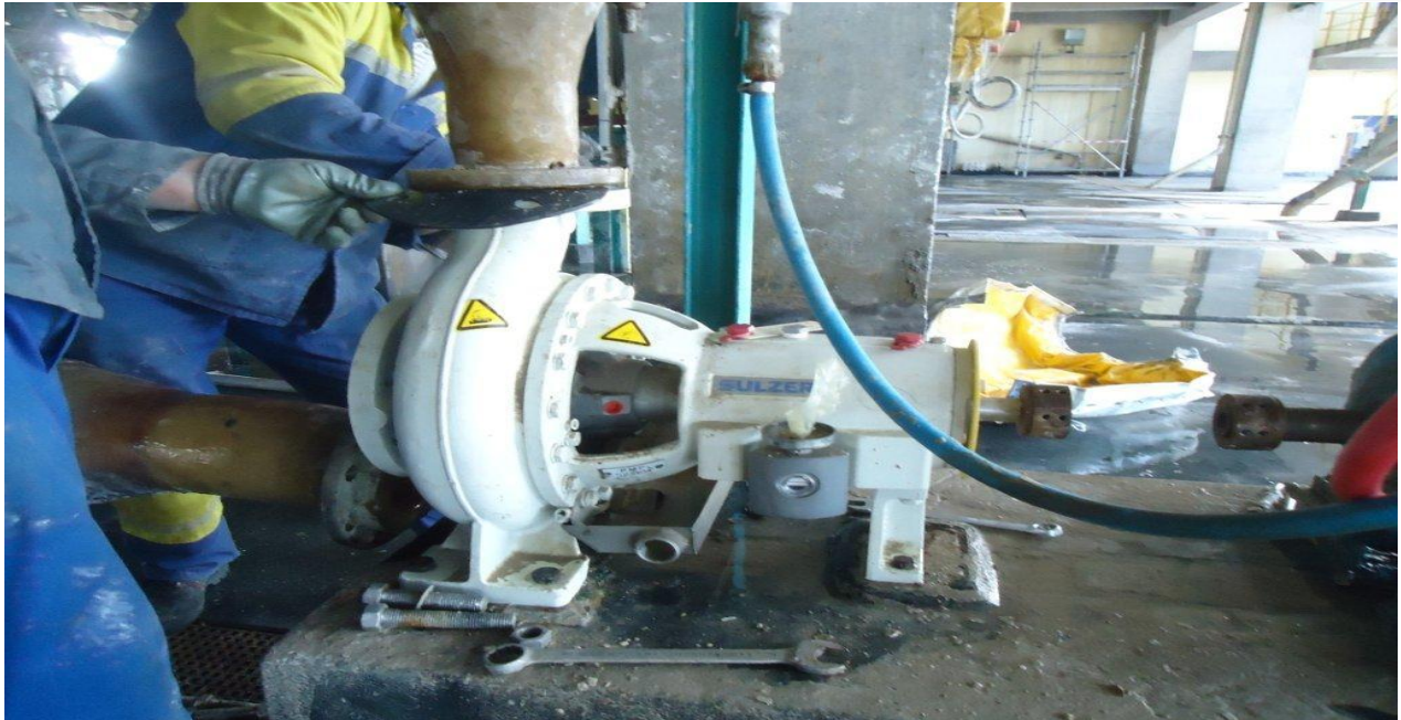
Figure 49: pompe centrifuge-PMP-AF-203AP36
