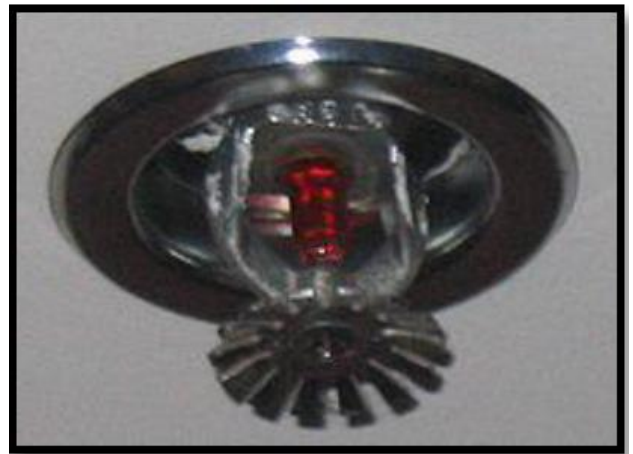
Figure 27: Splinkler
