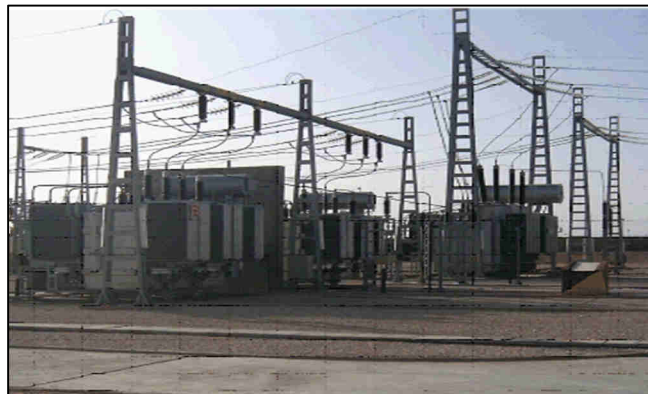
Figure 4 : Transformation THT/HT/MT
