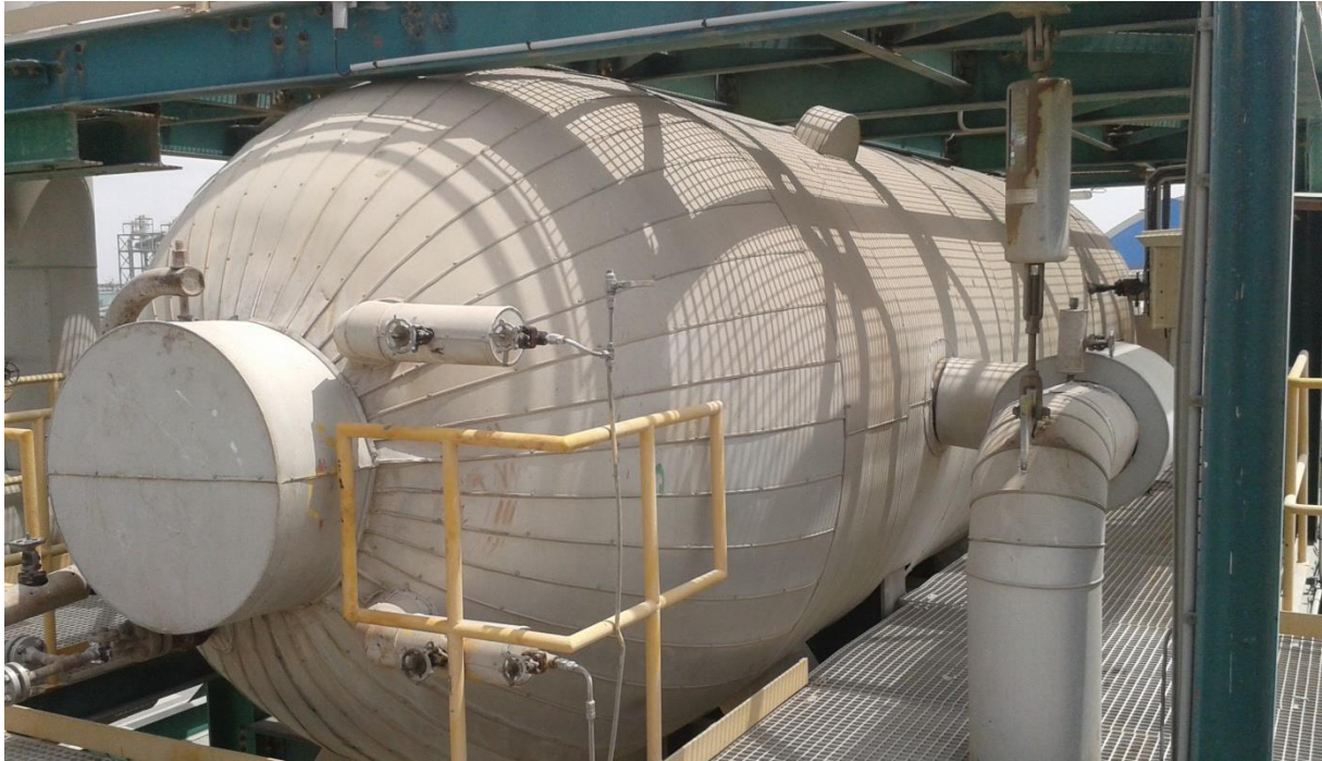
Figure I-2.3 Ballon de chaudière
