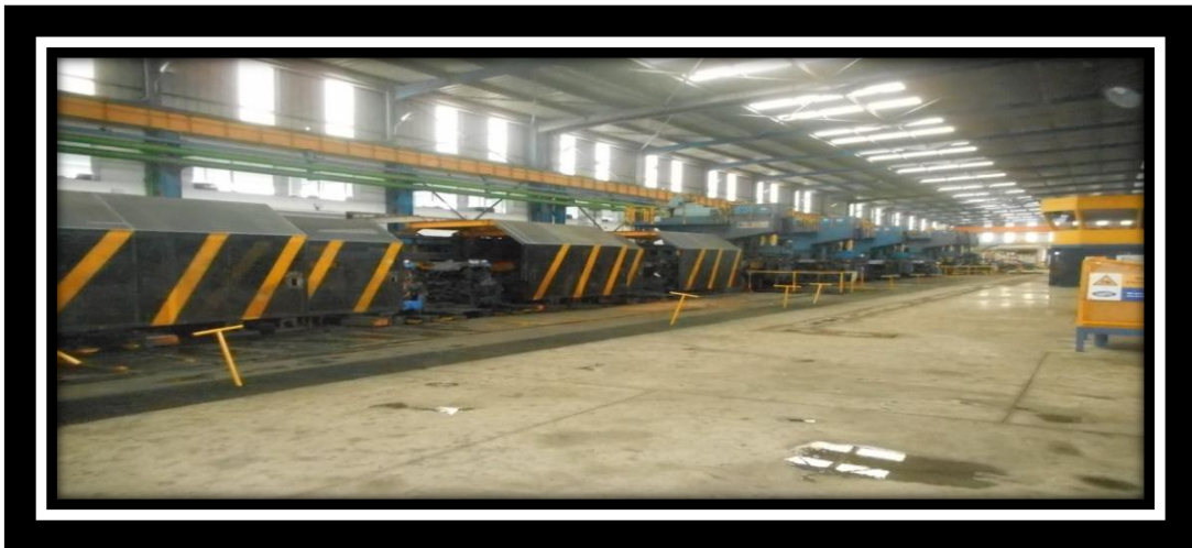
Figure 12: Train de laminage
