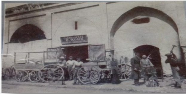
Figure 2: Construction des charrettes
