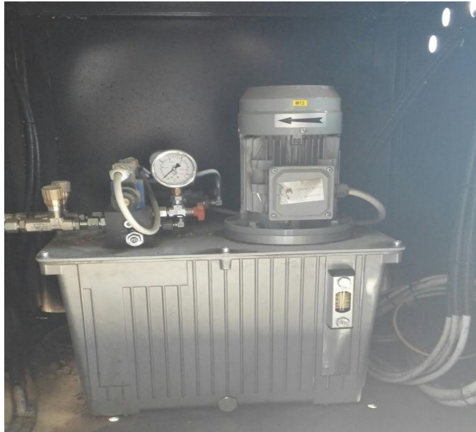
Figure 14 : Station hydraulique
