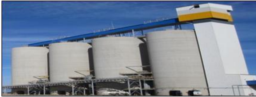
Figure 9: Silos de stockage du ciment
