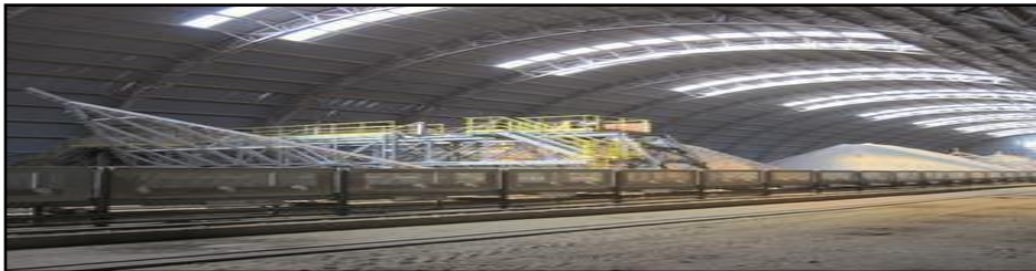
Figure 3:Les halls de stockage
