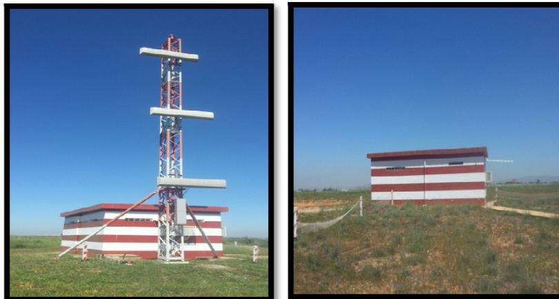
*Figure 6 : Station ILS : Glide Path+ DME-L+ Station Localizer*
