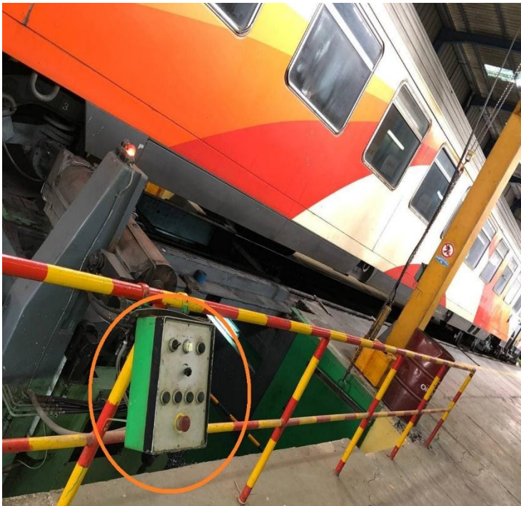
Figure 32: coffret de commande
