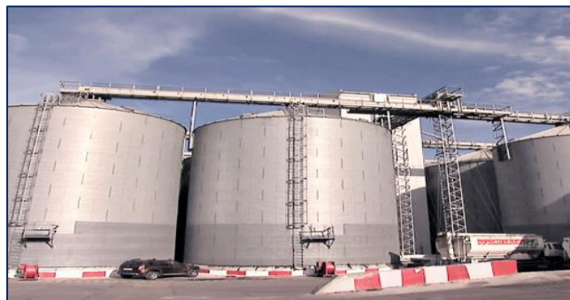
Figure 4: Silos de stockage
