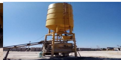
Figure 1.15: le silo de ciment
