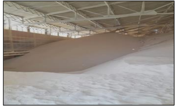
Figure 8: Zone de stockage de phosphate
