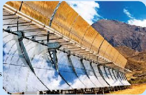
Figure 7: Centrale cylindro-parabolique [2]
