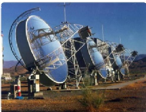
Figure 15: Installations de Dish-Stirling [3]
